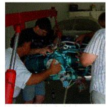
Figure 5. Aligning the Engine.
